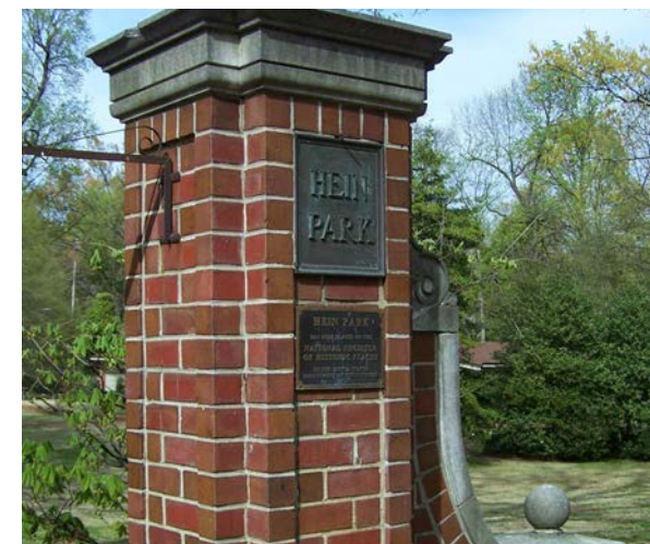
Figure 3.11 Brick piers with signage
